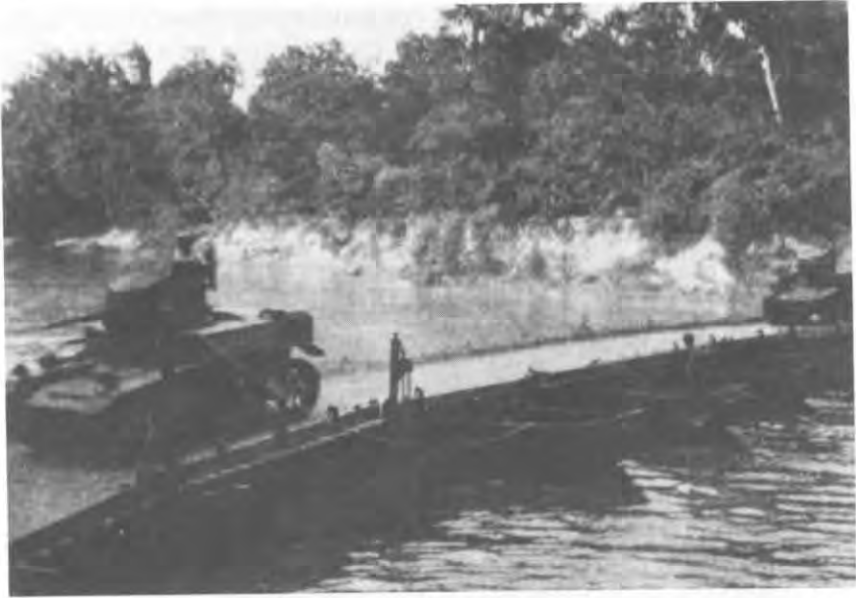
Light tanks cross the Red River on a Corps of Engineers ponton bridge. ( Armor magazine. )
